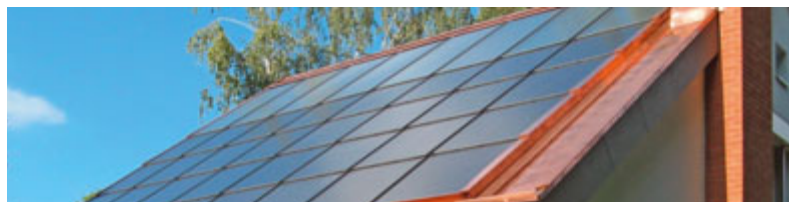
Photovoltaikanlage (Indach)
