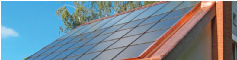
Photovoltaikanlage (Indach)
