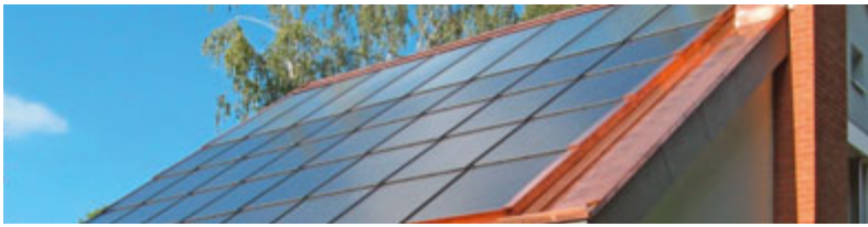
Photovoltaikanlage (Indach)
