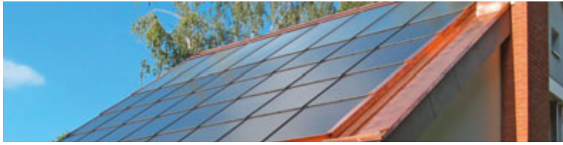
Photovoltaikanlage (Indach)
