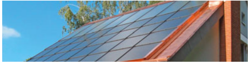
Photovoltaikanlage (Indach)
